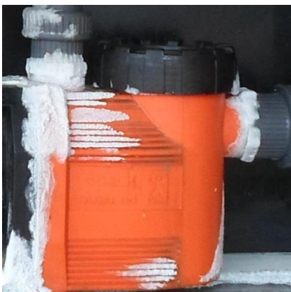
Inspect & repair pipework
