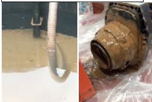
Tank not cleaned, pump failed
