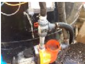
Bad leak at valve, potential pump problems
