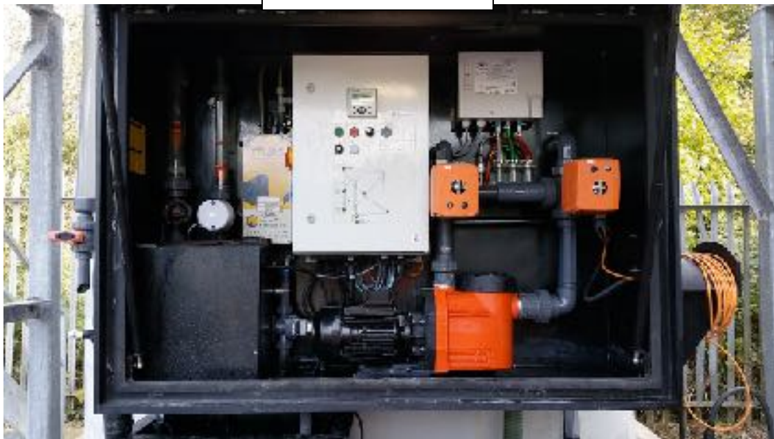
Serviced Pump Station
